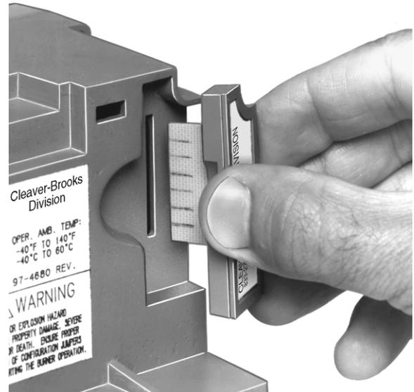
Fig. 11. Purge card installation.
