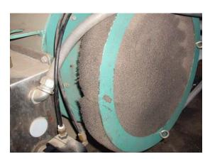
Problems can arise from blocked air filters if the burners go fuel rich; wasting fuel, dollars, creating carbon, and the potential for a fire hazard.
