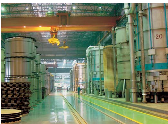
Fig. 7: LOI bell-type annealing installation
