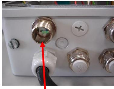
Fig. 16: Threaded insert of the EMC cable gland
