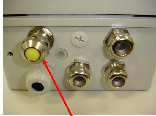
Fig. 14: Special EMC cable gland for installing the Ethernet cable
