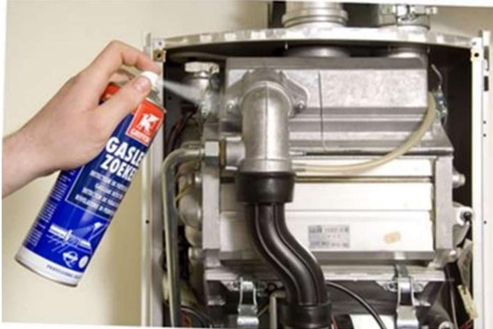
Figure 39. Aerosol detection agent made by Griffon
