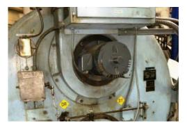
When the pilot and main flame are lit, immediately look for items such as the quality of the flame and the gas pressure stability entering the burner.
