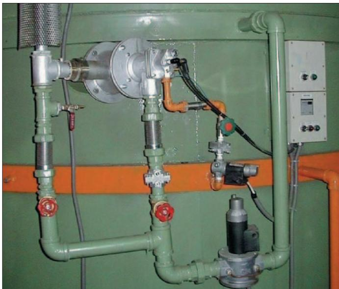
**Fig. 8:** Burner control
