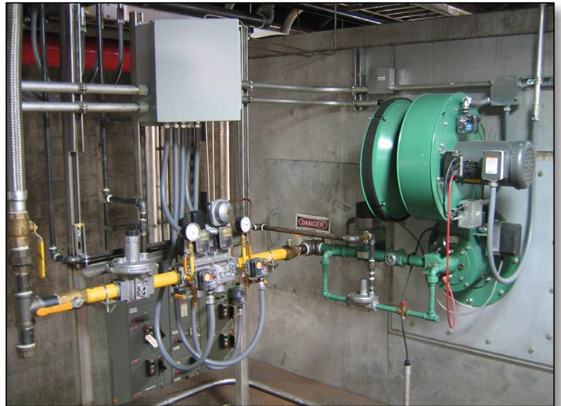
*Eclipse WX0300 installed with enhanced ratio control system*
