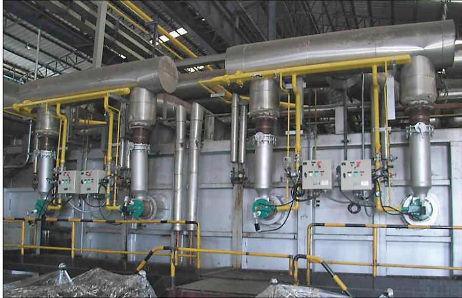
Pusher reheat furnace after burner conversion with TJPCA burners installed.
