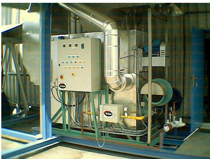
Recirculating Indirect Fired Air Heater
