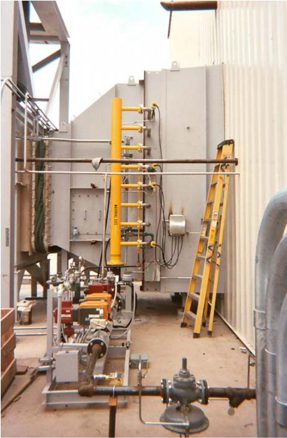
*Duct Burner with Inlet Transition.*
