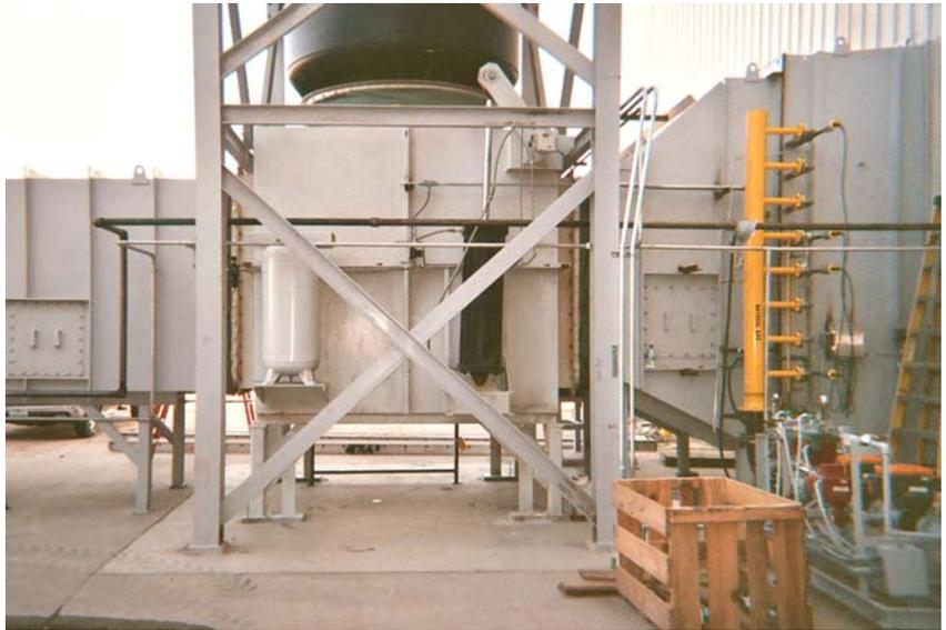
*Duct Burner Installed with Diverter Valve Upstream.*
