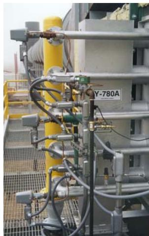
Detail of burner gas and air piping.
