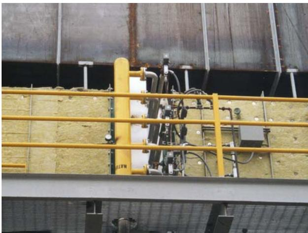
Burner installed in turbine exhaust duct.
