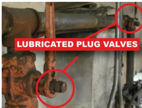
Lubricated plug valves seal by virtue of the sealant that is within them, if they aren't being maintained or lubricated with the correct sealant, gas may leak past the valve seat downstream into the fuel train piping or through the stem into the atmosphere.
