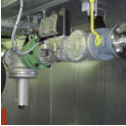
AVS works photograph
