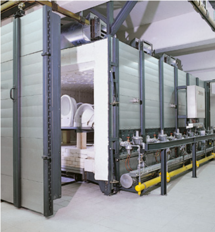
Ceramics kiln with temperature control via impulse system
