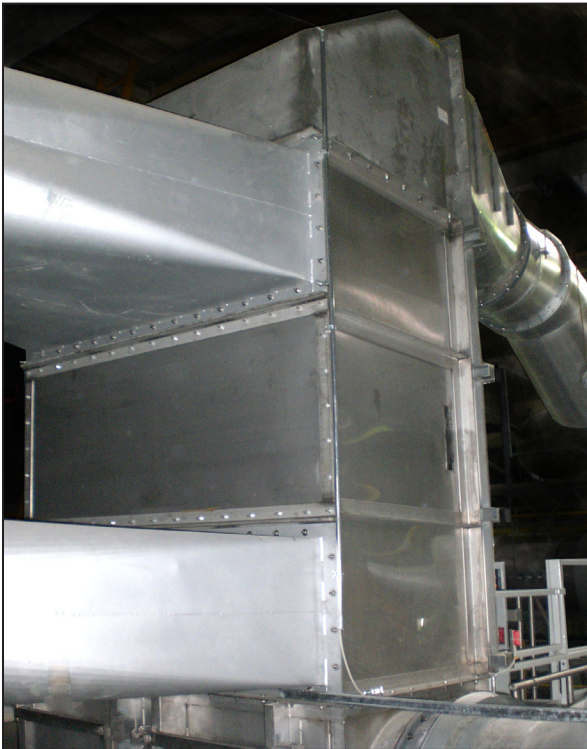
Heat Exchanger With Combustion Air Connection Ducts
