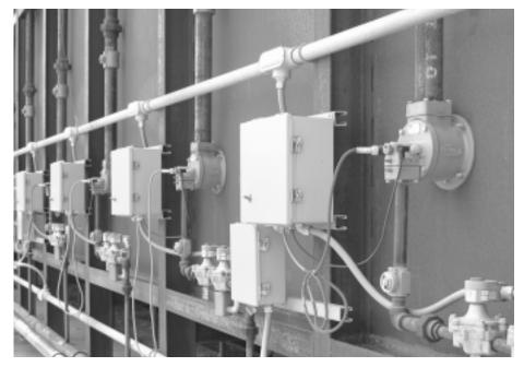
Effective post-weld heat treating for stress relief plays a crucial role in the quality and reliability of SRS Wintergreen's processing equipment. For the new car-bottom furnace, the company selected Eclipse ThermJet burners to provide efficient, uniform and environmentally superior process heating.
