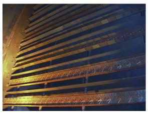
Burner installed in duct
