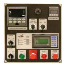
The integrated annunciator significantly reduces troubleshooting downtime compared to conventional panels without limit annunciation. An LED flame signal indicator is provided as standard equipment.
