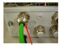
Fig. 17: Fitted EMC cable gland
