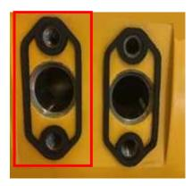
Figure 35. Thickness of paints should comply with tolerance and specification 0.25mm+0.25
