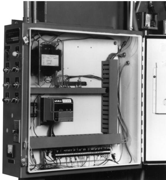
**Fig. 11. Electrical Panel installation.**
