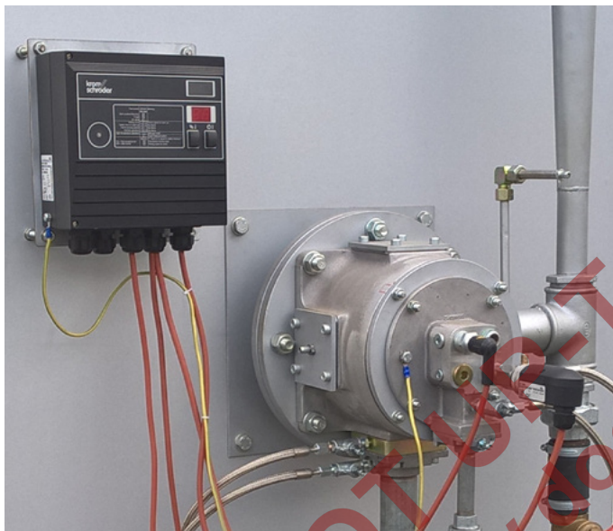
ECOMAX burners with burner control unit BCU
