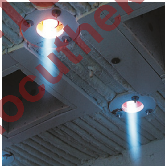
Overhead firing with BIC burners
