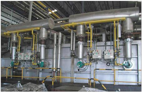
Pusher reheat furnace after burner conversion with TJPCA burners installed.
