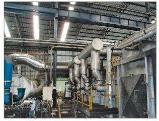
Pusher reheat furnace before burner conversion.
