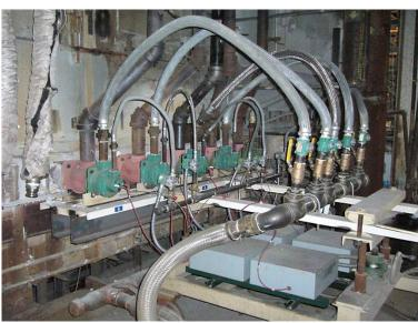
Overall view of edge heating system installed on tin bath.
