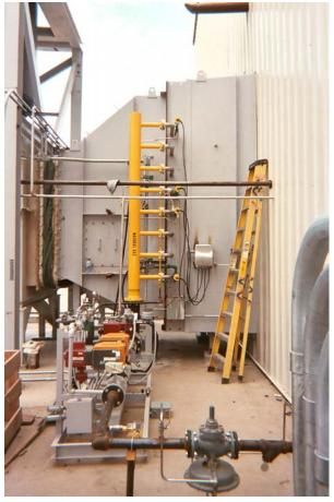
Duct Burner with Inlet Transition.
