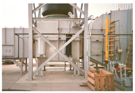
Duct Burner Installed with Diverter Valve Upstream.
