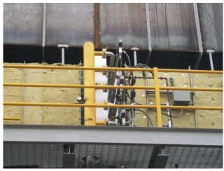
Burner installed in turbine exhaust duct.
