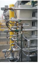
Detail of burner gas and air piping.
