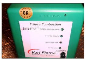
All repaired units are marked with our gold **MODIFIED OK ECLIPSE** stickers. These are also good to use and have been converted to the new design.
