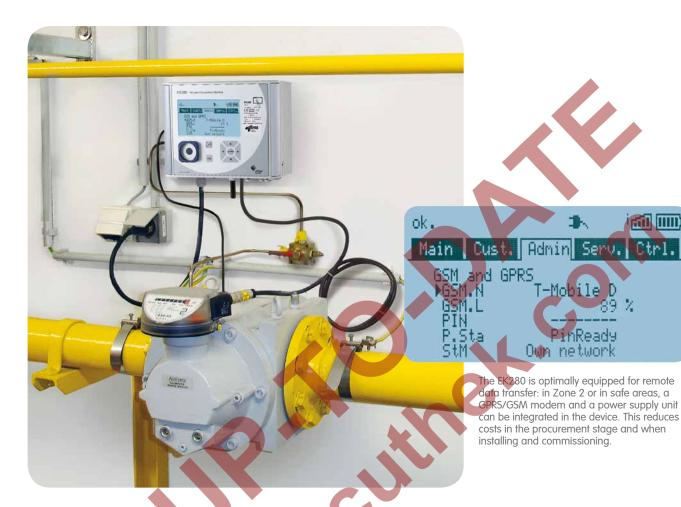
In short – the EK280 is multilingual and in addition to its "mother tongue" IEC 62056-21, it is equally "fluent" in the Modbus protocol and DLMS/COSEM communication. What is more, if in future new requirements should emerge for communications, so that so-to-speak new "vocabulary" is needed, or if something changes
