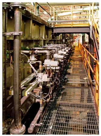
This large scale conversion is easily balanced due to symetrical pipework. (34) ignition transformers and (34) UV flame detectors.
