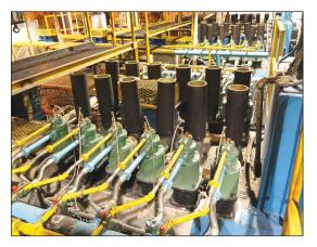
After: By converting the furnaces from SER v1 to SER v5 burners, the customer was able to save time and money and lower their  $NO_X$  emissions.
