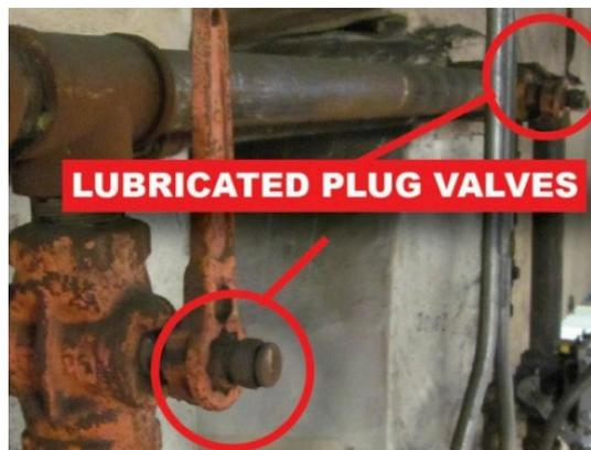
Lubricated plug valves seal by virtue of the sealant that is within them, if they aren't being maintained or lubricated with the correct sealant, gas may leak past the valve seat downstream into the fuel train piping or through the stem into the atmosphere.
