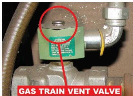
Incorrectly vented gas train components including vent valves, regulators, pressure switches, and relief devices also may allow for a release of gas into the workplace atmosphere.
